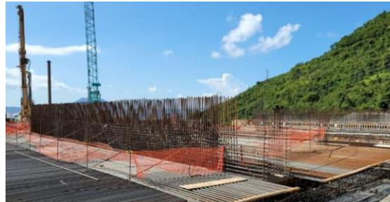
Construction of base slab of service reservoir
