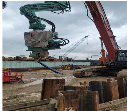
Noise mitigation measures on sheet piling works
